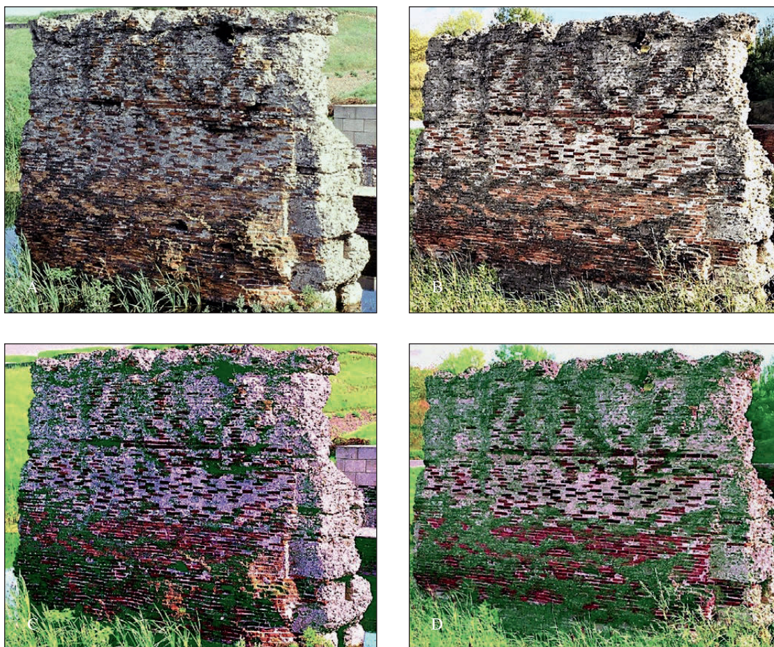
Fig. 4. Biocolonisation on the northern side of the pillar: in the period from the late 1980s to the 1990s (A) (Archive of the Institute of Archaeology), and in 2020 (B) (Archive of the MoDeCo2000 project); from the late 1980s and 1990s (C) and from 2020 (D); images enhanced using DStretch app (RGB0) (Archive of the MoDeCo2000 project)
