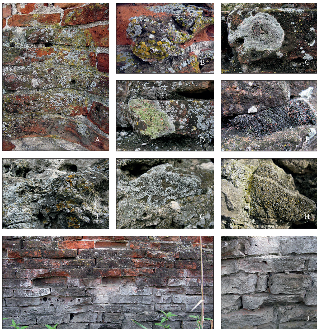
Fig. 6. Lichen and moss infestation of brick (A–D), mortar (E), and stone (F–H) of the pillar in September, 2022; lower, usually submerged part is discoloured and infestation free (I–J) (Archive of the PROTECTA project)
