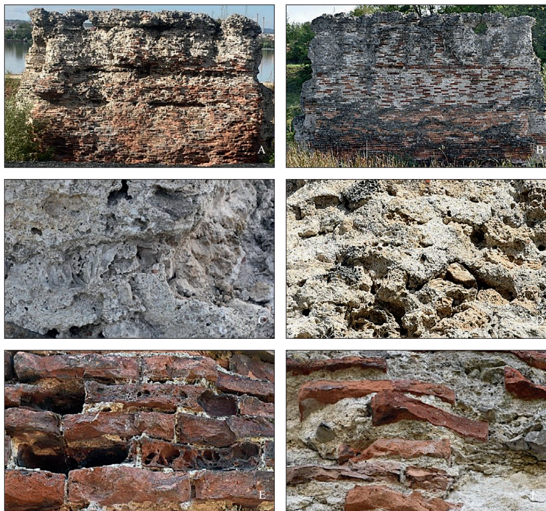
Fig. 5. Deterioration of the pillar – southern side in 2020 (A), and northern side in 2022 (B); stone and mortar deterioration in 2020 (C, D); brick and mortar deterioration in 2021 (E), and in 2022 (F) (Archive of the MoDeCo2000 project)
