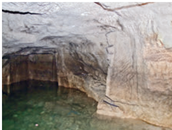
Fig. 12. Perfectly preserved traces of quarrying in the upper gallery
