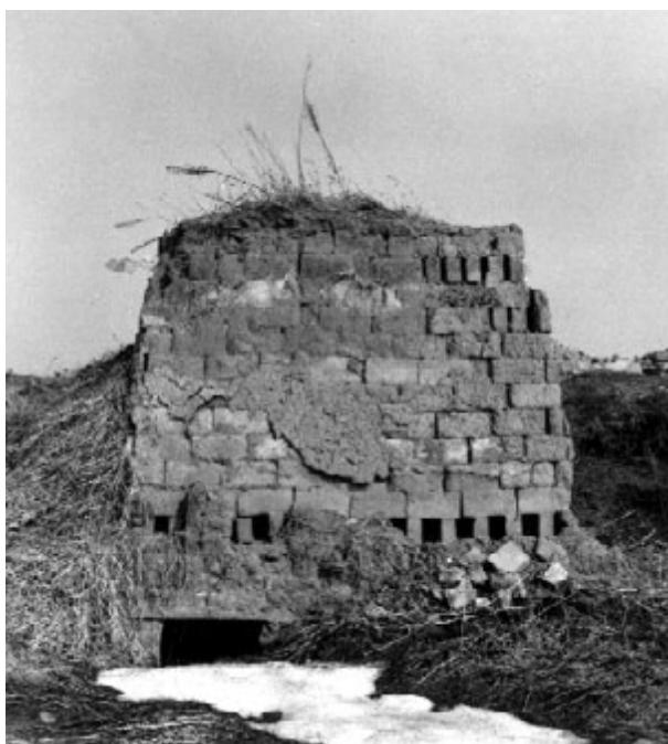
*Fig. 34. Brick kiln in the Požarevac area. Upper chamber is replaced by a clamp of dried bricks set edgewise. All visible surfaces are coated with a mixture of clay and chaff (photo M. Jeremić)*
