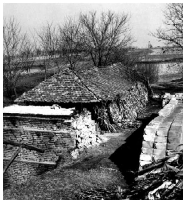
*Fig. 33. Semi-sunken roof tile kiln in the Požarevac area in the firing phase of the process. It is topped with a thick clay coating. In background: dried tiles stacked under a long roof, a kiln load ready for firing (photo M. Jeremić)*
