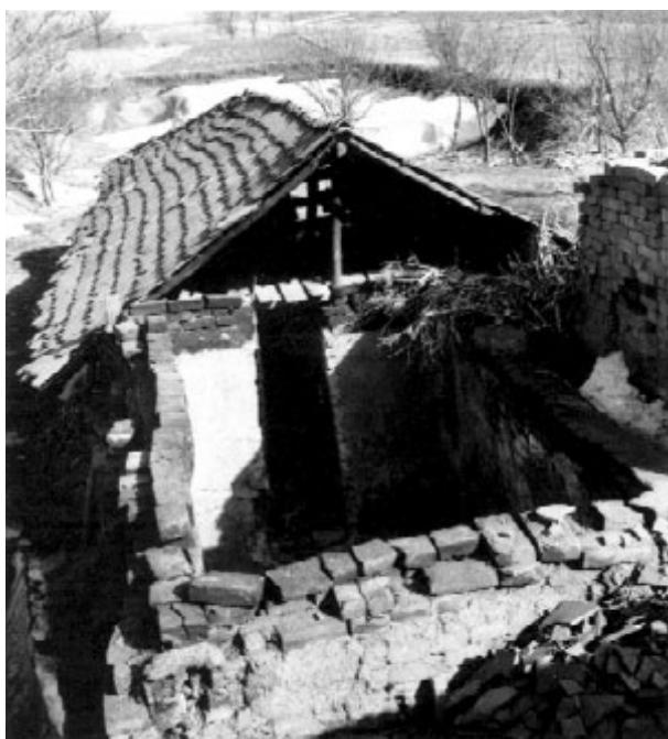
*Fig. 32. Brick and roof tile kiln within a private brickyard in the Požarevac area. Clearly discernible on kiln wall, in background: entrance to upper chamber (photo M. Jeremić)*
