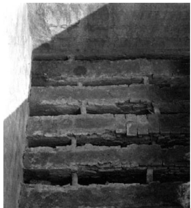
*Fig. 31. Bird's-eye view of brick-built cross walls in a sunken brick and roof tile kiln on a private estate in the Požarevac area (photo M. Jeremić)*
