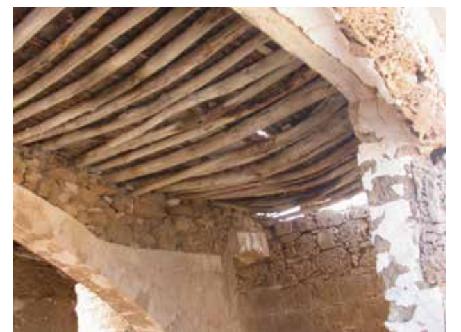
Fig. 7 - Roof construction with wood support poles and branches, covered with a layer of plaster, between the roof support stone arches. (photo D. Safrai)
