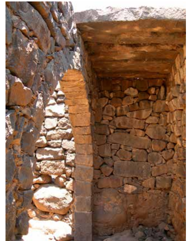
Fig. 6 - Roof Construction with stones, in Corazin, Galilee. This was the system of roofing also in Gamla. (photo D. Safrai)
