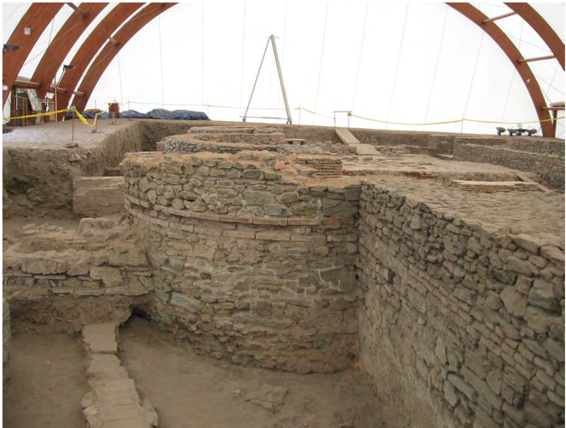
Fig. 32 Opus incertum mixtum in the walls of Viminacium thermae. Photo documentation of the Project Viminacium, Archaeological Institute Belgrade.
