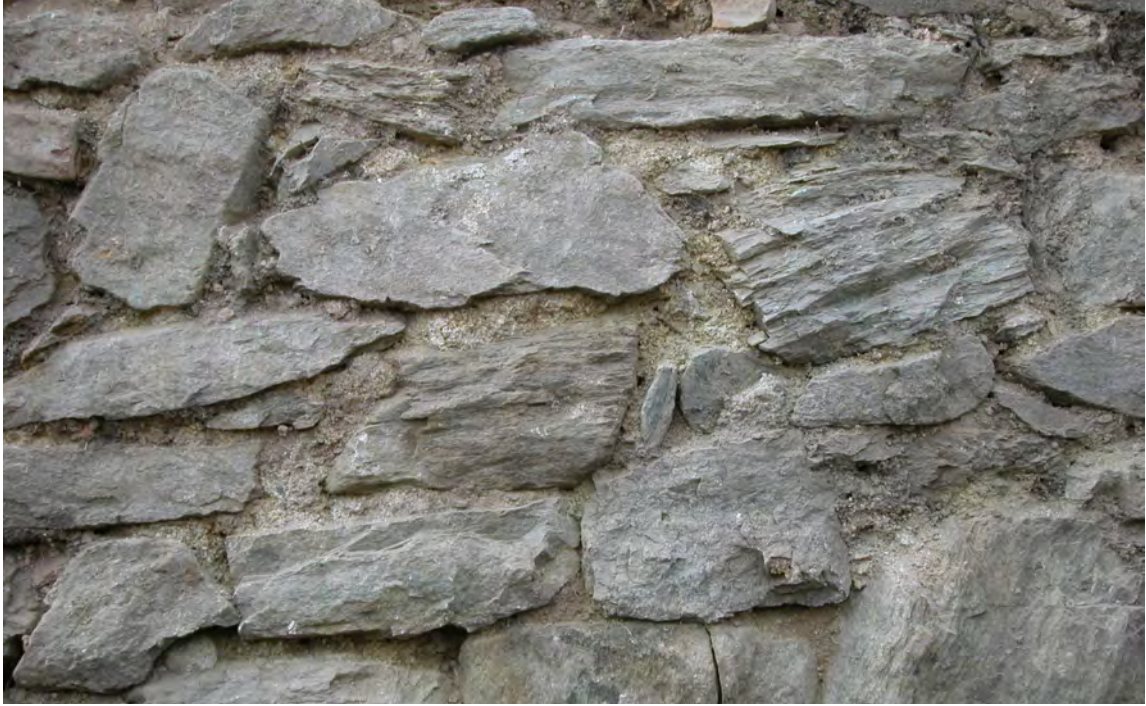
Fig. 31 Opus incertum in the walls of Viminacium thermae. Photo by the author.
