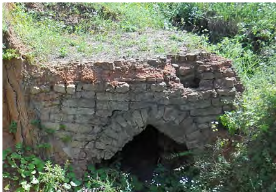
Fig. 13 Brick kiln built of adobe. Photo by the author.
