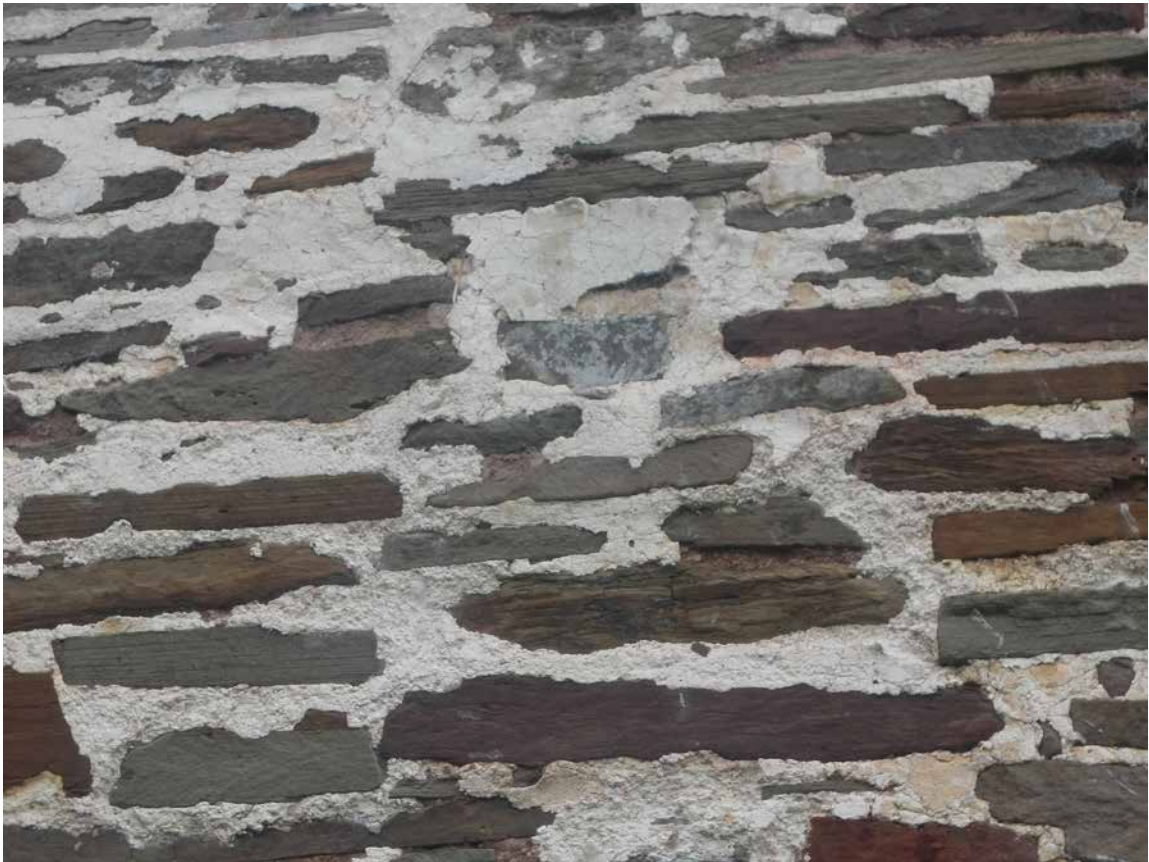
Figure 15. Church of St Clydawg, Clodock, Herefordshire. Very long in situ lime and hair pointing mortars over pit sand bedding mortars, as well as remnant of limewash surface treatment (photo taken by Nigel Copsey).
