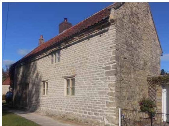
Figure 8. Spring View Farmhouse, Pickering, North Yorkshire. Repointed by the author in October 2024 with a dry slaked, hot mixed pointing mortar, 1.5 non-hydraulic slaked lime: 0.5 fine limestone dust: 0.5 sand and hair. Note the dryness of the repointed facade compared to the gable end wall still, at this time, with its cement pointing (photo taken by Nigel Copsey).
