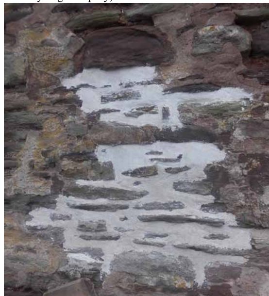
Figure 20. In situ lime and hair pointing trial by the author for English Heritage/Historic England, Longtown Castle Keep, Herefordshire, built with clay-sand mortars c1220 (photo taken by Nigel Copsey).
