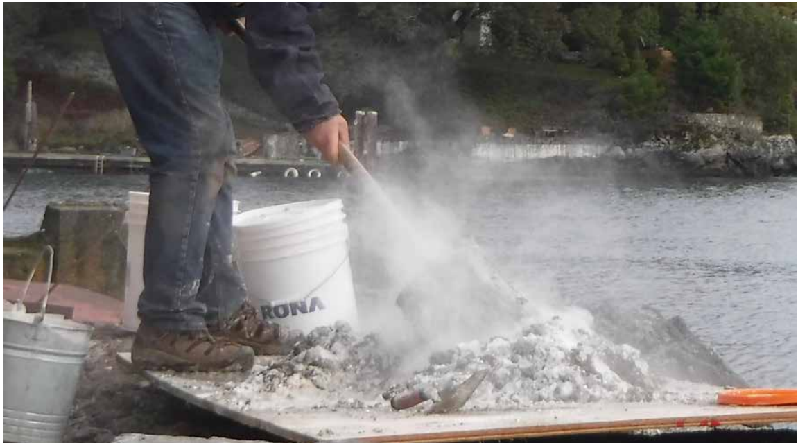
Figure 2. Turning and wetting a dry slaked mortar made using the ‘ring of sand’ method (photo taken by Nigel Copsey; Copsey 2019a: 150; Copsey 2022: 215, Figs. 19–22).
