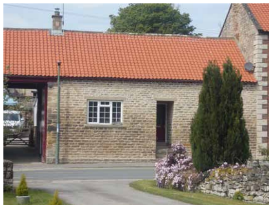
Figure 9. Calcareous sandstone building repointed in November 2023. Fabric saturated by long-term cement pointing. Within 2 days of completion, and regularly through the winter, overnight temperatures fell to minus 10 and minus 15°C. Mortar ratio 1 lime: 1 sand, dry slaked. No frost damage (photo taken by Nigel Copsey).
