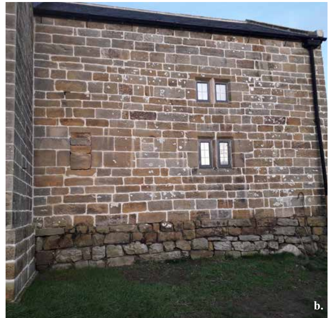
Figure 16. a. Lime and hair (only) plaster onto sandstone masonry, 17 th century building; b. its exterior recently repointed with a hot mixed lime mortar, North Yorkshire Moors (photos taken by Nigel Copsey).
