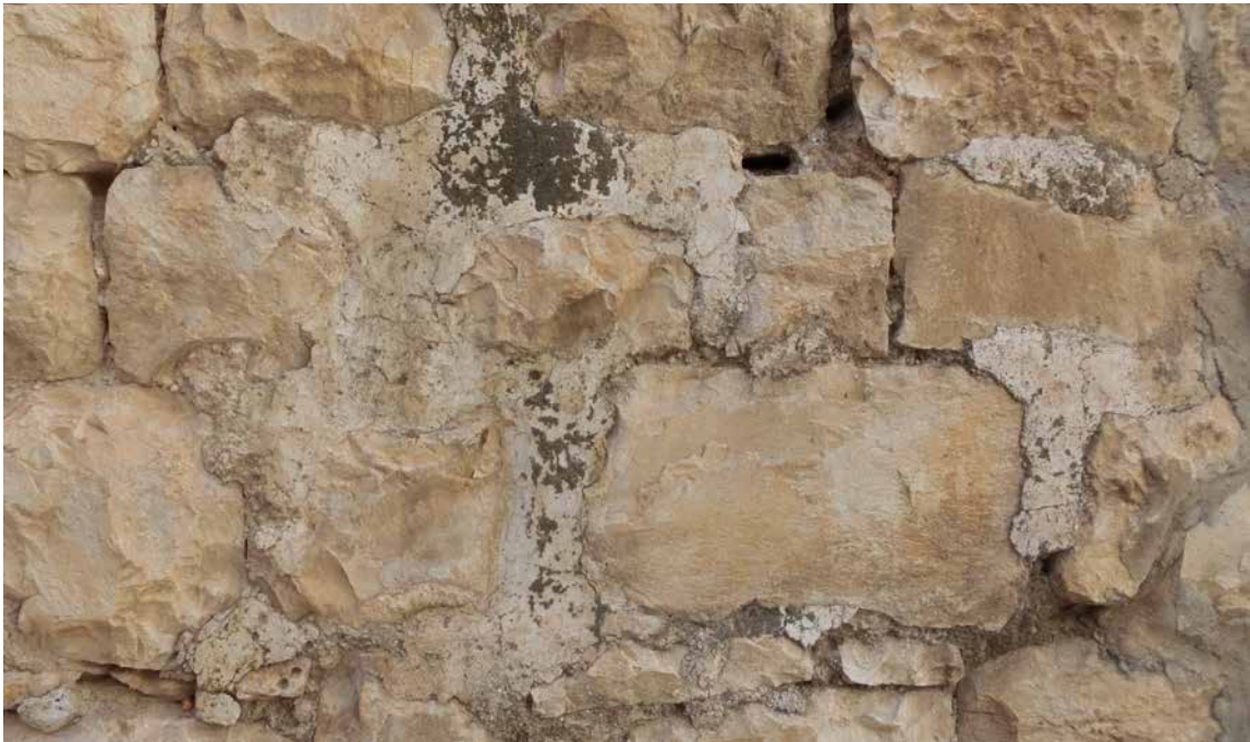
Figure 13. Lime only mortar over earth lime bedding mortars, Akko (Acre), Israel. On analysis by Bill Revie, this was of non-hydraulic lime only and without even fibre. Dry slaked, but used after cooling (photo taken by Nigel Copsey).
