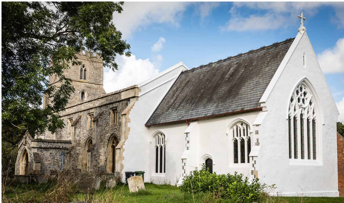
Figure 21. Reinstatement of lost hot mixed lime renders and limewashes, West Wrating, Cambridgeshire. Not only historically authentic and drying of the fabric but providing a carbon sink (photo taken by Ashley Courtney and published with his permission).
