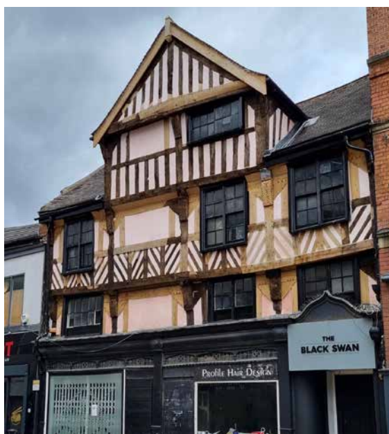
Figure 10. Circa 1610 timber framed building, Wakefield, West Yorkshire. Repaired in 2023 by the author and timber-framer Wayne Kirby. Infill panels and internal plasters, like-for-like dry-slaked lime and hair plasters, finished with hot limewash (photo taken by Nigel Copsey).
