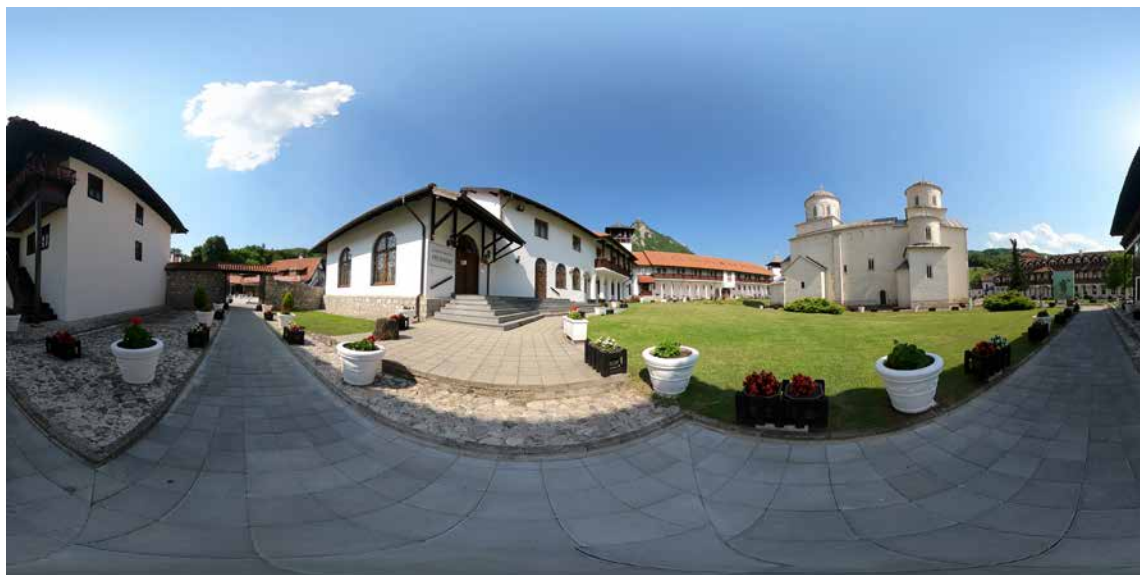
Figure 7. Mileševa Monastery, 360° photo in Flat view mode (photo by the authors, 2022).
