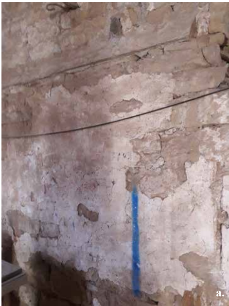
Figure 16. a. Lime and hair (only) plaster onto sandstone masonry, 17 th century building; b. its exterior recently repointed with a hot mixed lime mortar, North Yorkshire Moors (photos taken by Nigel Copsey).
