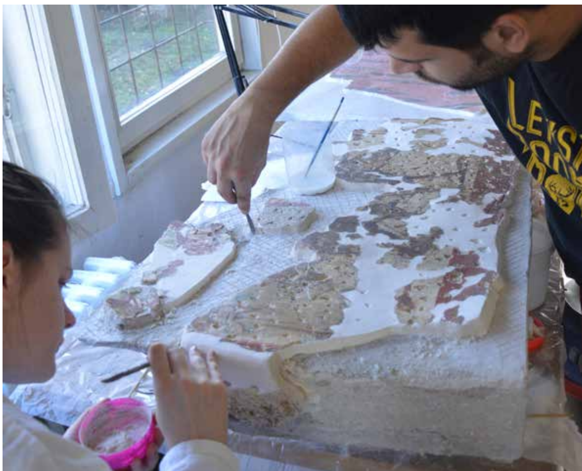
Figure 5c. Construction 1 - Conservation of wall painting from the earlier phase (photo by the author).
