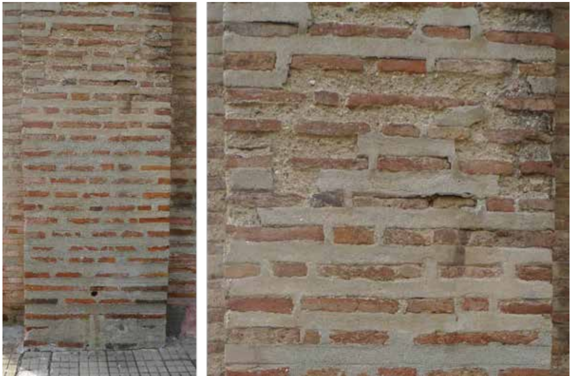
Figure 4. Problematic interventions with cement-based materials (photo by the author).
