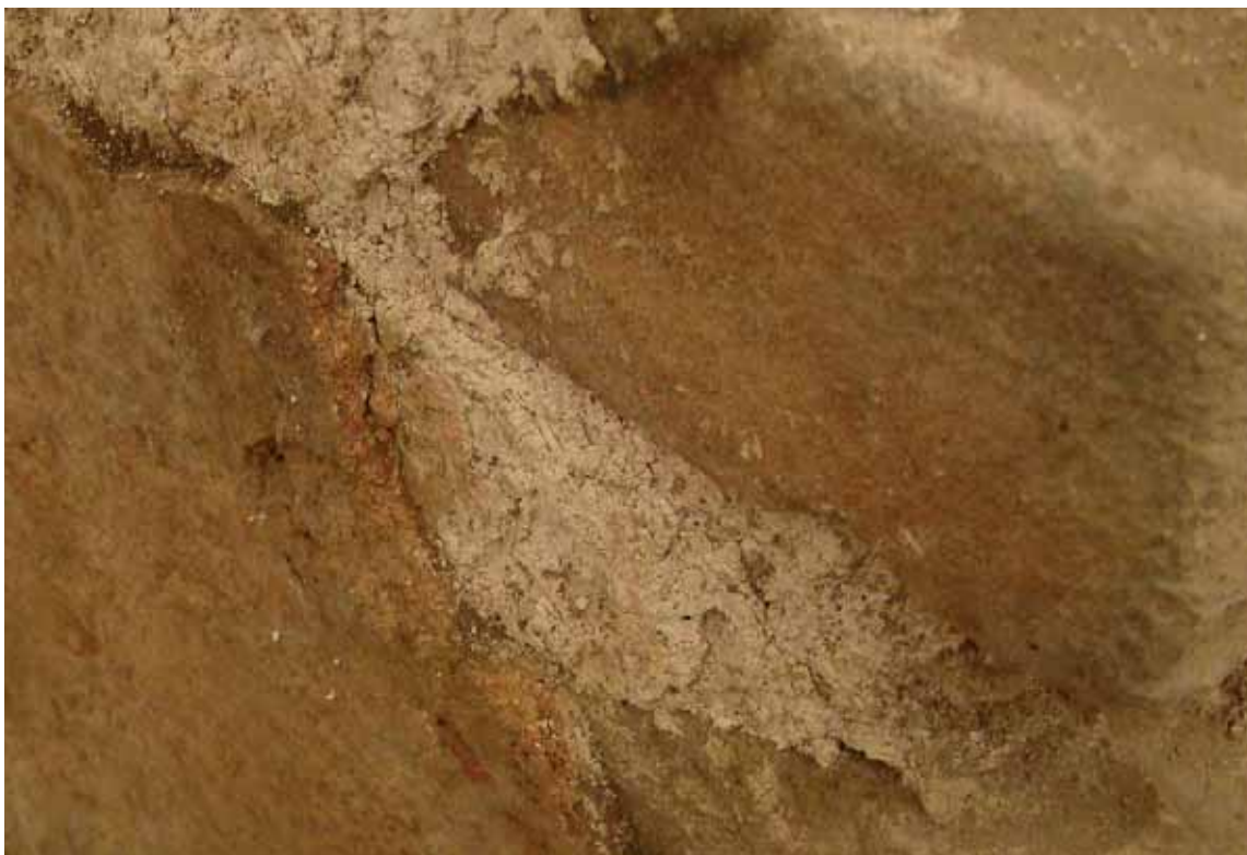
Fig. 14 Rendering layers of Viminacium thermae with brick in the form of small fragments and in the form of a dust. Photo-documentation of Institute of Archaeology Belgrade
